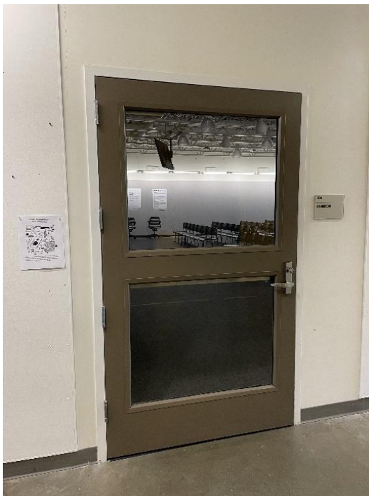
Image Description: Two-windowed door looking in to Arch 104.
