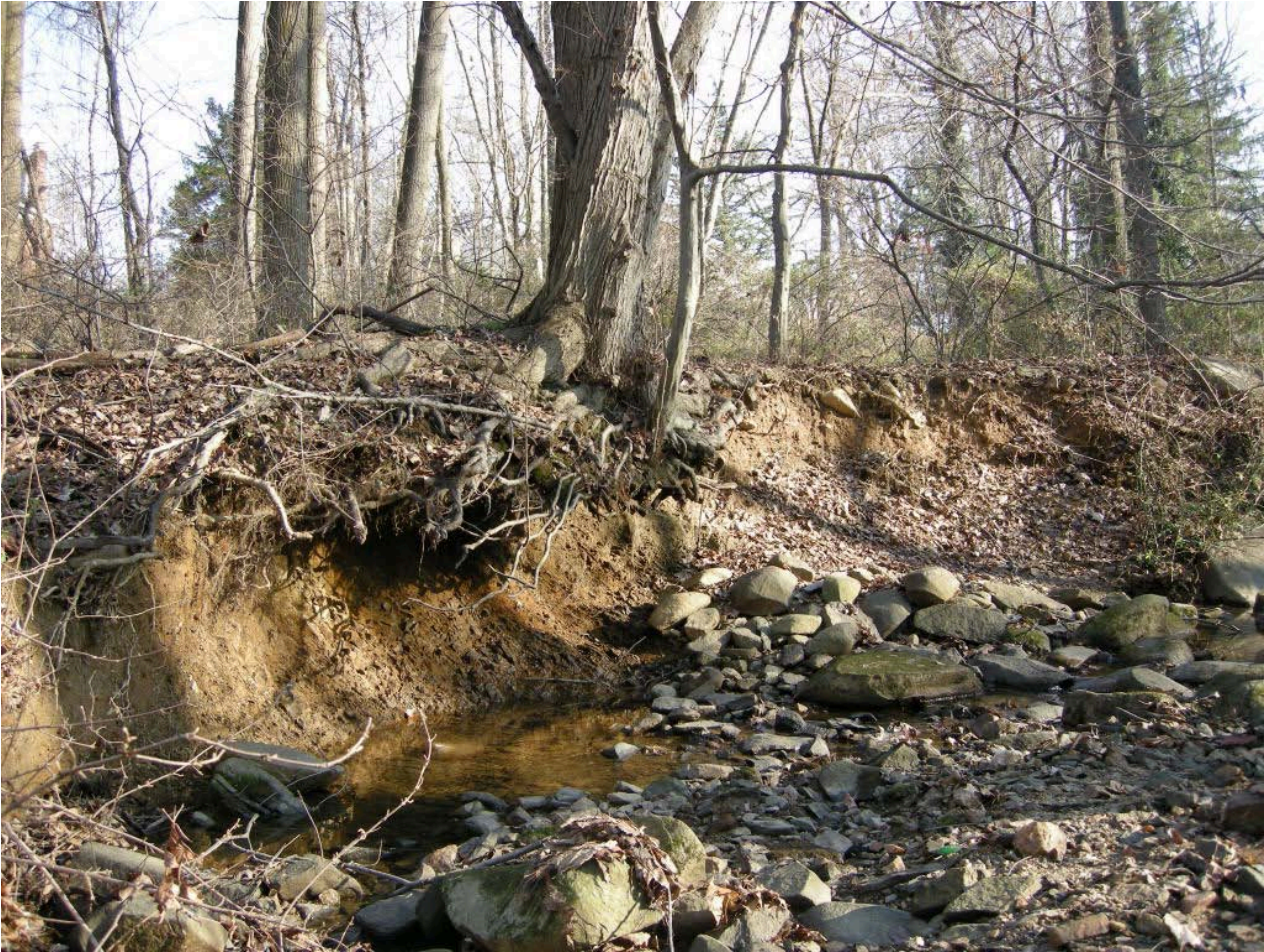
Figure 3.2.B Example of streambank erosion and bank undercutting tributary to Pennypack Creek, Lower Moreland Twp., Montgomery County, PA
