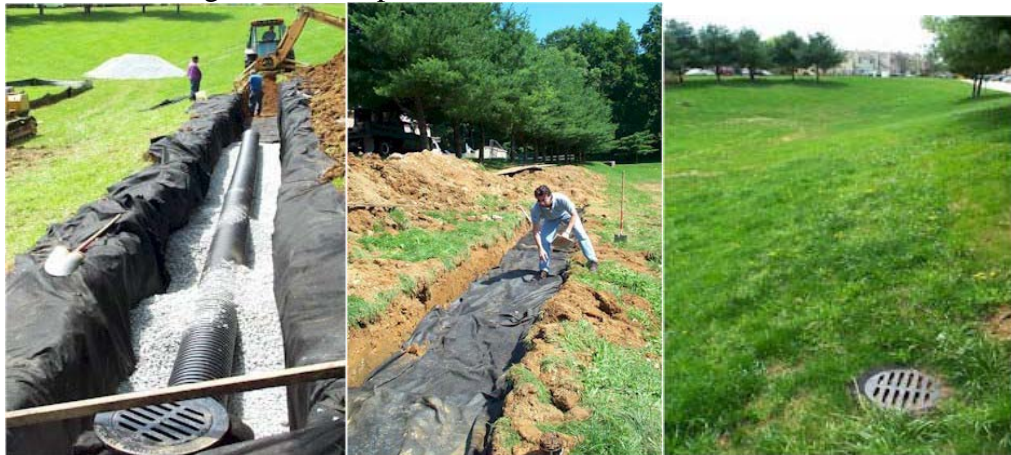
Figure 3: Example of Infiltration Trench Installation
