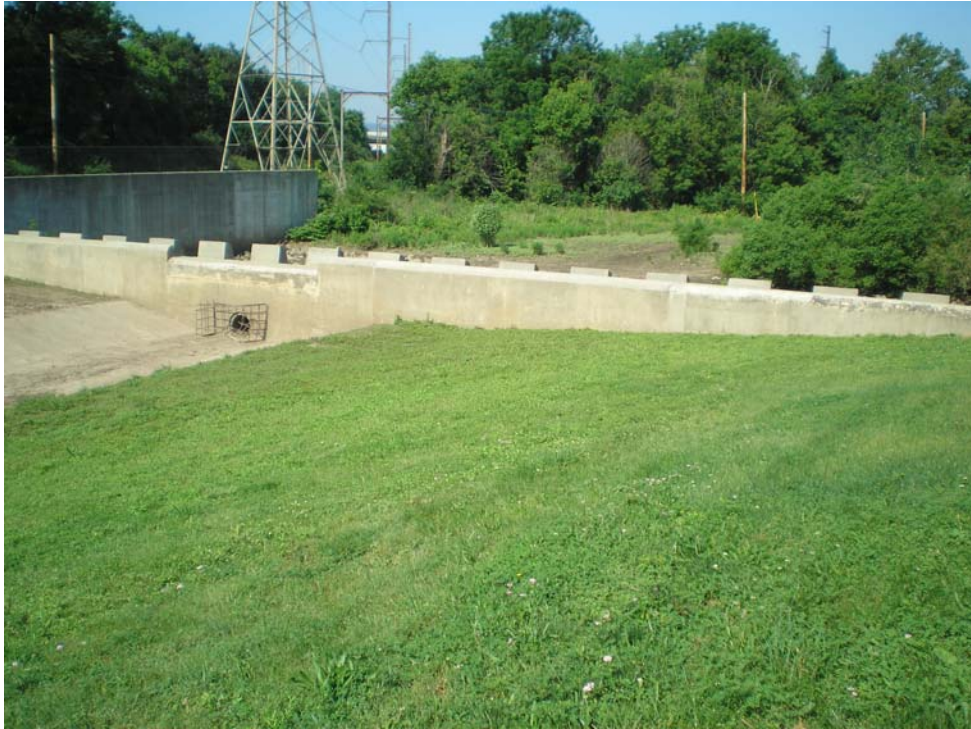
View facing downstream, note base-flow pipe at center of dam's upstream face
