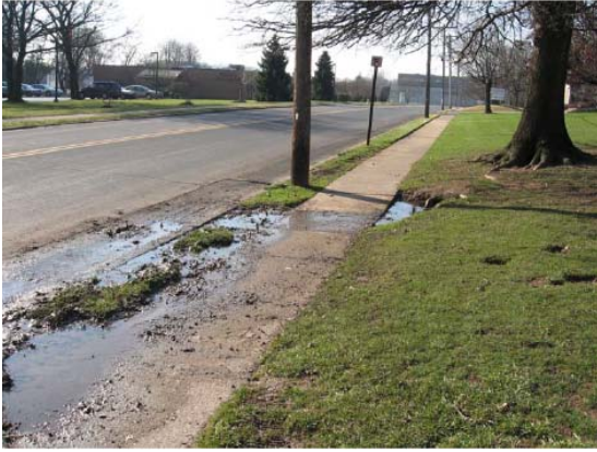
Curb failure – New York Drive
