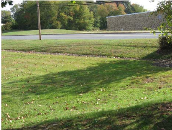
Swale and infiltration trench – New York Drive
