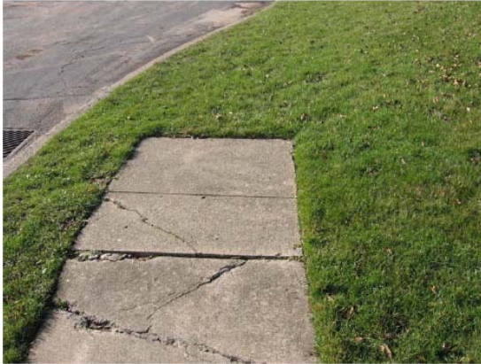
Cracked sidewalk to nowhere – New York Drive
