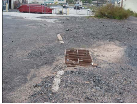
Battered storm drain – New York Drive
