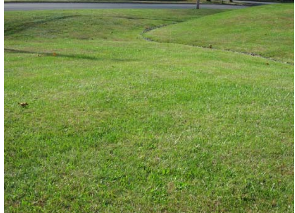
Swale and infiltration trench – Maryland Drive
