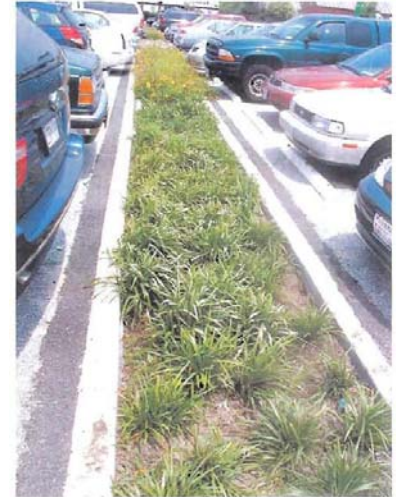
Lined Bioretention Strip in parking area
