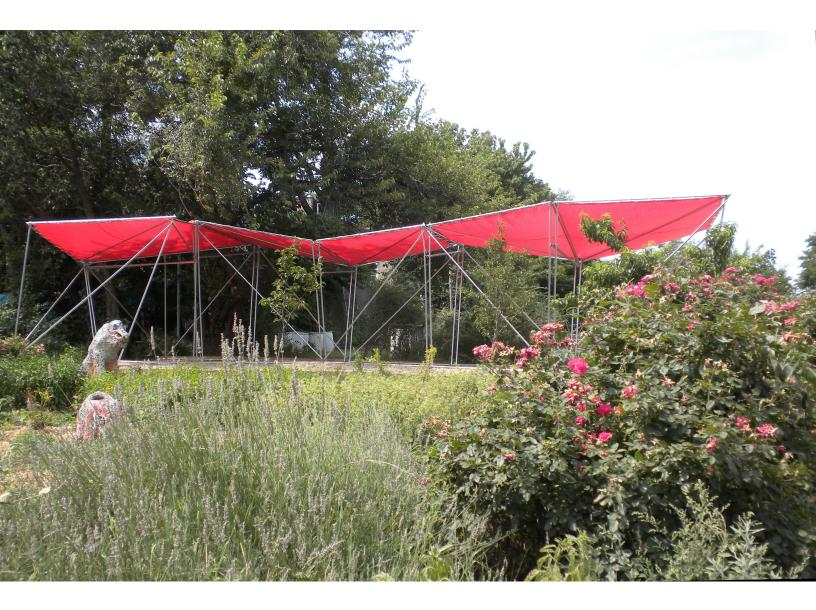
Project Description: The pavilion serves as shade structure and teaching space for the urban gardening program at Philly Earth. Built in modules with simple materials, it can be moved and reconfigured according to programmatic needs.
