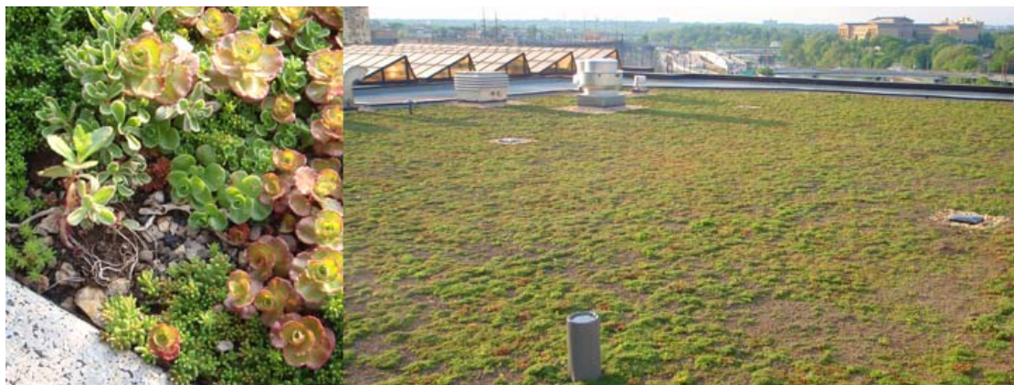
"Green Roof" Courtesy of Philadelphia Water Department
