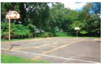
8. Court surface is poor and cracked surrounded by overgrown vegetation.
