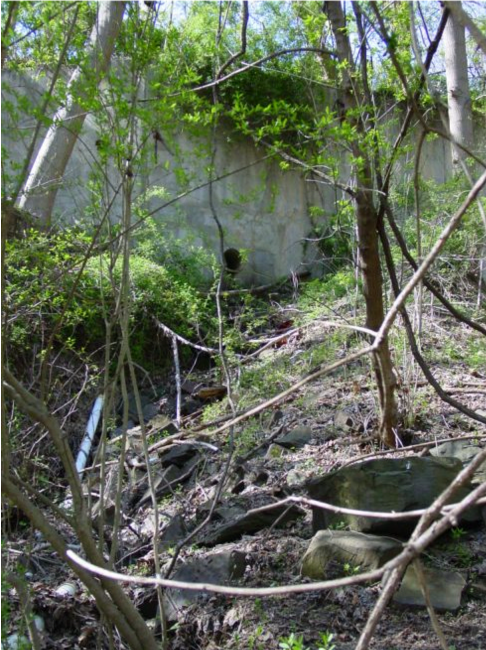
Figure 2a: Stormpipe L1 in Abington Township, which discharges through Lorimer Park.
