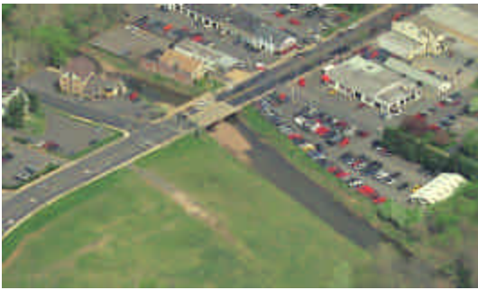
Figure 11: Rapid urbanization in the floodplains is common throughout the Pennypack Watershed
