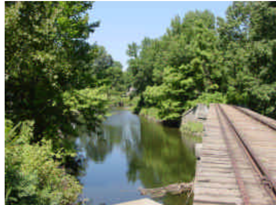
Figure 3: A railroad bridge crossing the main stem of the Pennypack Creek
